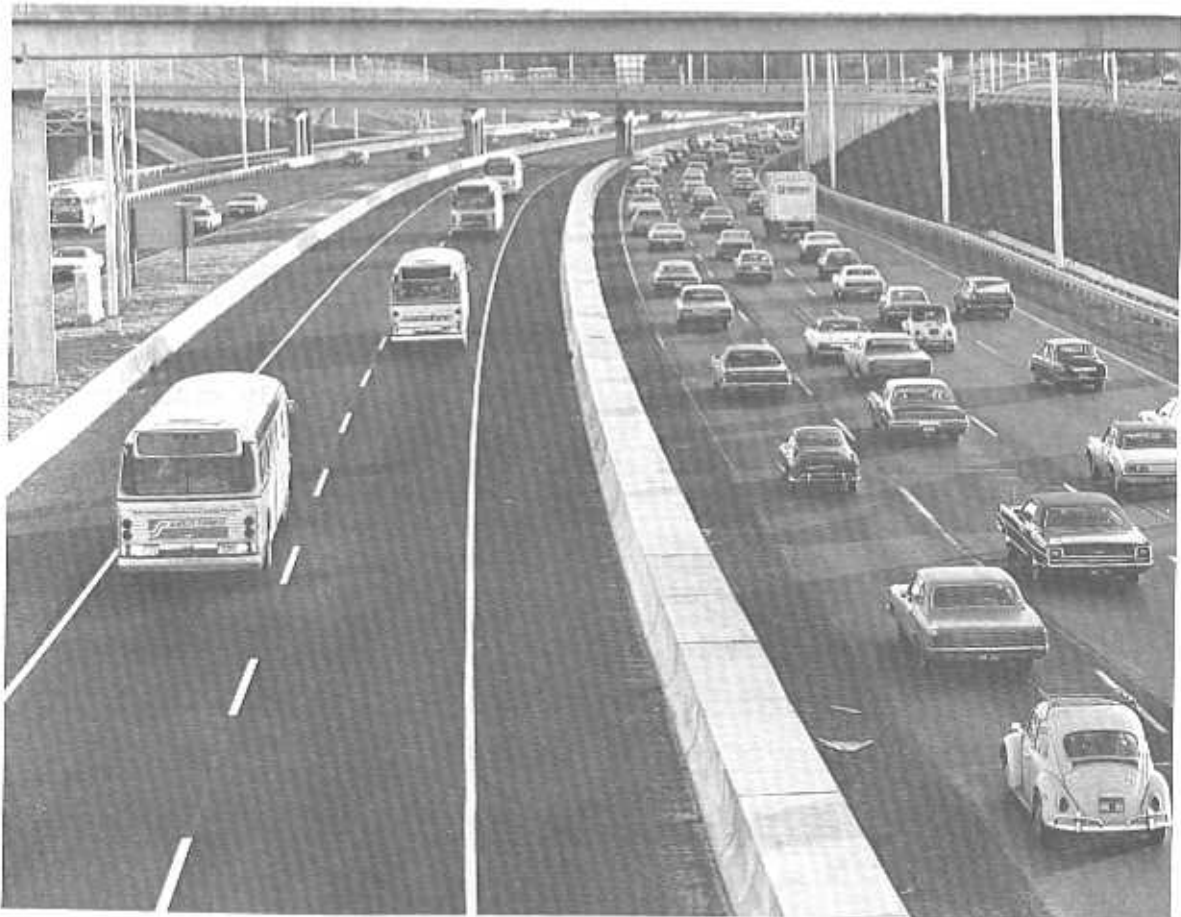
The increased people moving capacity of the exclusive bus lane is demonstrated in the above photo.
