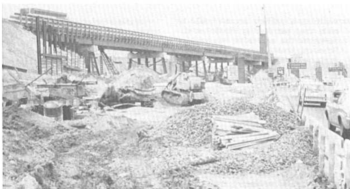
An express bus travels over the temporary roadway bridge.
