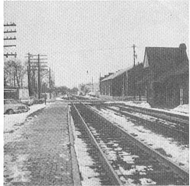
⑭ Gaithersburg (B&O) Looking West. Storage Track to Left in Distance
