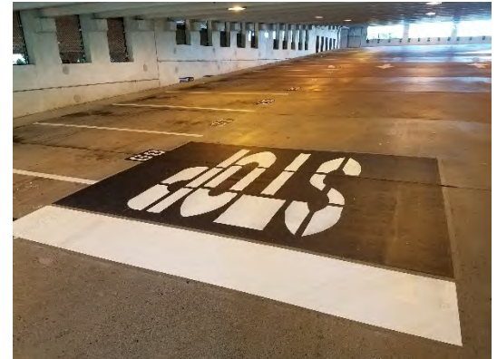
Manassas Station Garage Striping (after)
