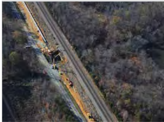
An existing water culvert under the CSXT main line is being widened as part of the HA-XR Third Track Project in order to support the new track.
