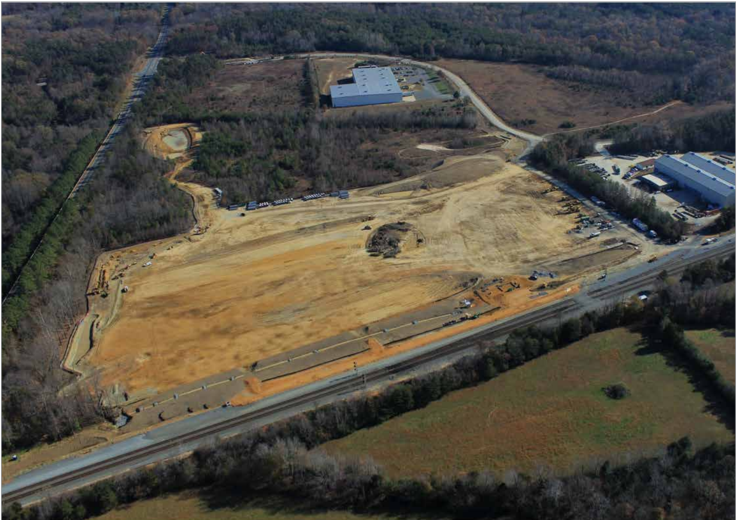
Spotsylvania County has extensively cleared the area needed for the new parking lot while VRE contractors proceed in the foreground with the construction of the platform and spur track serving the new station
