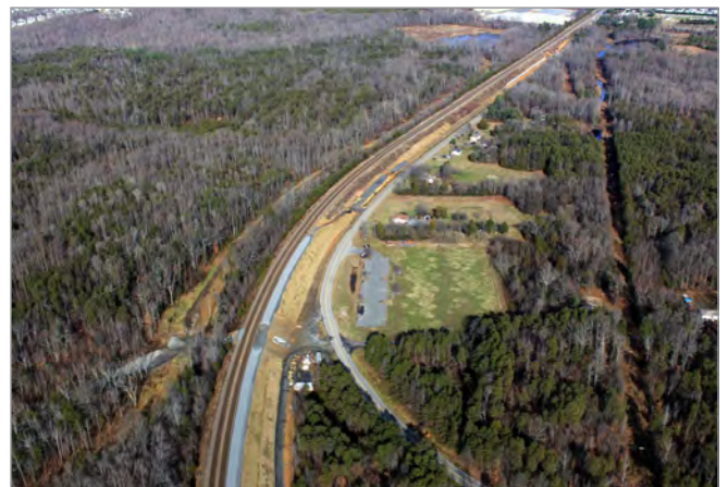
Ballast is being laid for the third track roadbed heading northward alongside Benchmark Road in Spotsylvania County prior to the installation of the new track.
