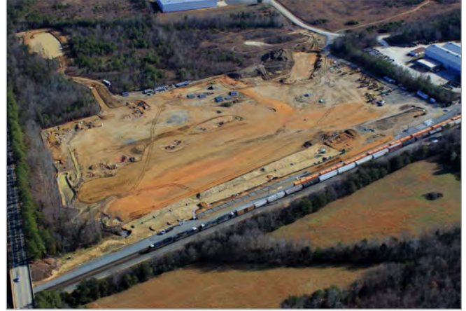
CSXT freight trains run past the worksite for the new Spotsylvania Station. VRE's contractor is working on new track and platforms in the foreground while the County's contract or works on fill and drainage for the parking lot.
